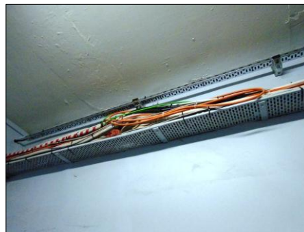
PHOTOGRAPH 14 TYPICAL VIEW OF CABLING ON HIGH LEVEL CONTAINMENT ACROSS BASEMENT AREAS
