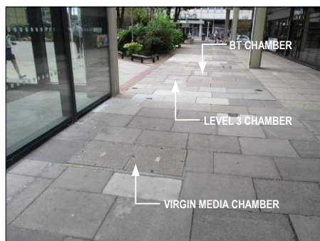
PHOTOGRAPH 1 EXISTING BT, LEVEL 3 AND VIRGIN MEDIA CHAMBERS IN FOOTWAY AT NORTH WEST CORNER OF BUILDING
