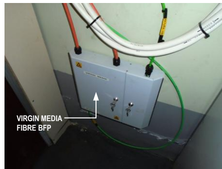
PHOTOGRAPH 11 VIRGIN MEDIA BUILDING FLEXIBILITY POINT ON WALL BENEATH BT COPPER DP
