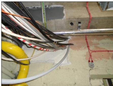
PHOTOGRAPH 13 TYPICAL VIEW OF SERVICES FROM PRIMARY INTAKE IN TANK ROOM EXITING AT HIGH LEVEL TOWARDS RISER
