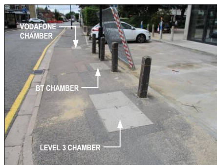
PHOTOGRAPH 2 EXISTING LEVEL 3, BT AND VODAFONE CHAMBERS IN FOOTWAY ON DUKES AVENUE TO SOUTH ELEVATION OF BUILDING
